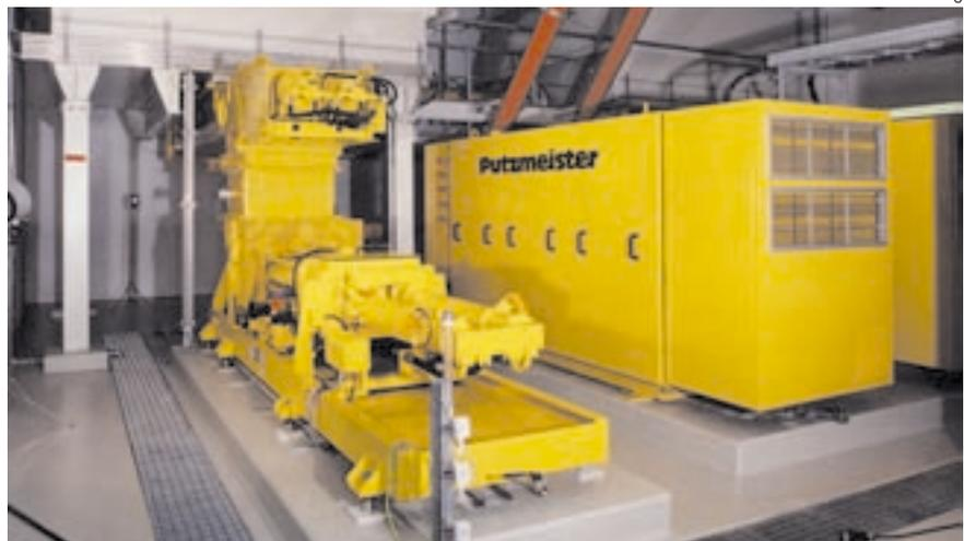
Co-incineration of sewage sludge in the coal-fuelled power station Zolling: solids pump KOS 2180
