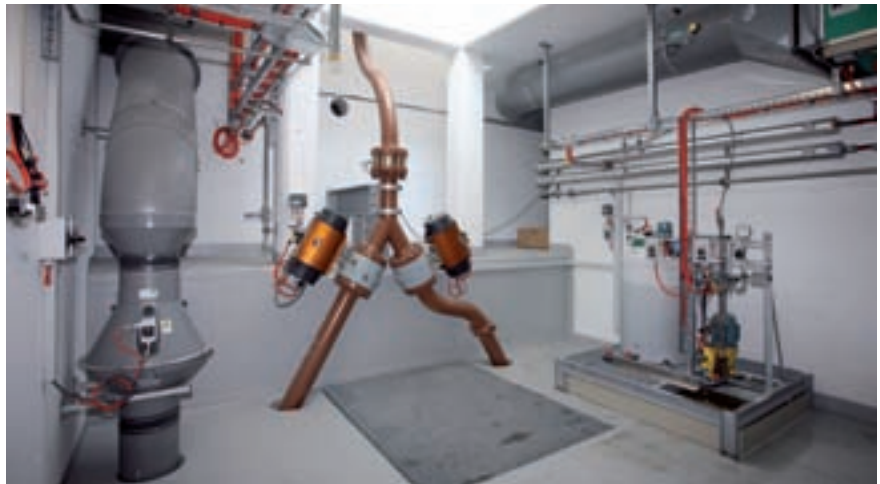
BLI – injection unit for lubrication of the pipeline if pressure loss is rising
