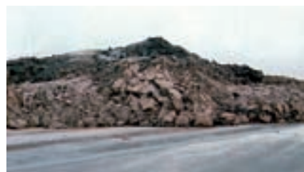
The sludge with lime has a solids content of about 40%. It is distributed over a wide area by the Geysir method.
