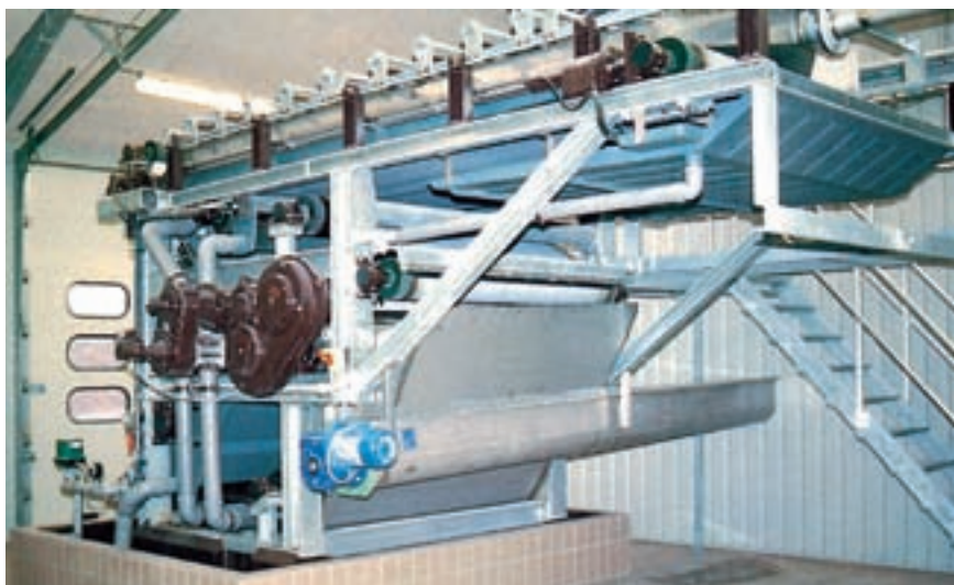
View of the filter band press. A shaftless auger conveyor for sludge passes through the wall
